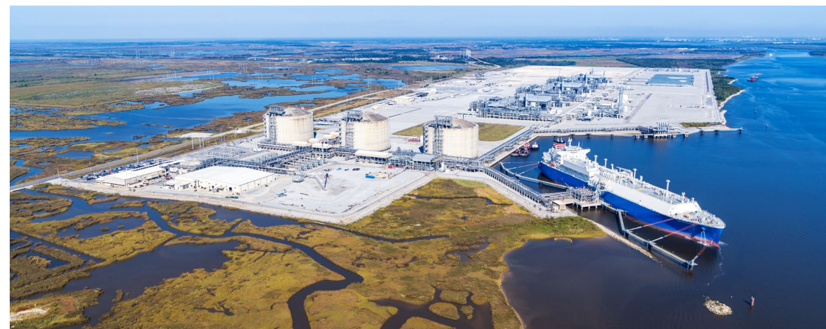
The LNG Enterprise carrier being loaded at the Cameron LNG liquefaction terminal in Louisiana. © Cody Porche - Porche Aerial Imagery - TotalEnergies
