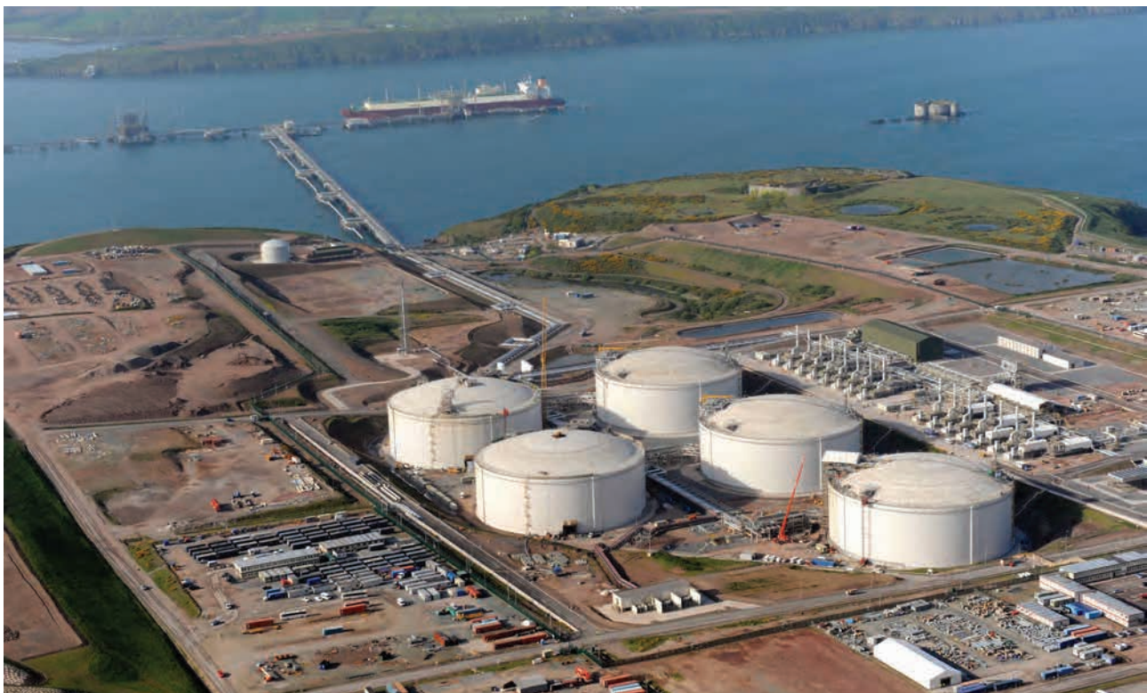
South Hook regasification terminal.
